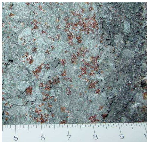
Fig. 11 View of half of a vertically sawn sample
