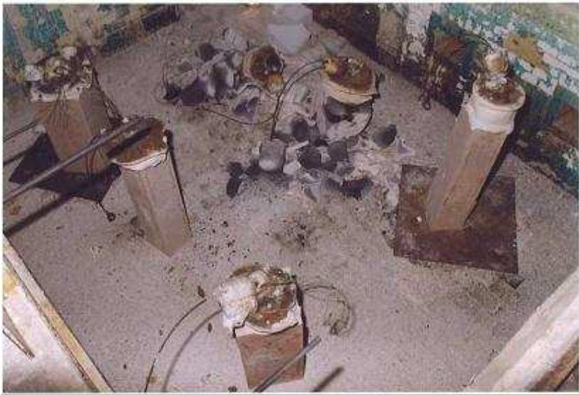
Fig. 8 The 6 columns made with Ductal® after ISO Curve Fire tests; the picture clearly shows that no spalling or slight spalling was observed on the columns made with Ductal® -AF, the 2 other columns made with Ductal®-FO were completely destroyed and fell down
